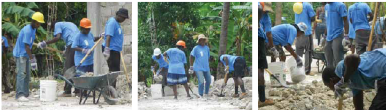
A work crew clears rubble from a home outside Léogâne, Haiti.
